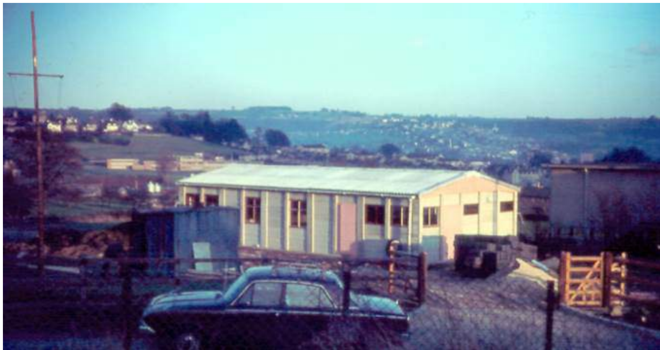
HQ under construction.
